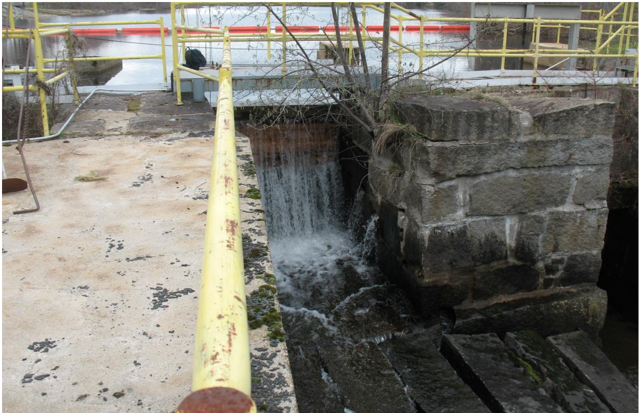
Photo 14. Downstream View of East Sluice. Note Leaking Stoplogs and Trees in Masonry.
