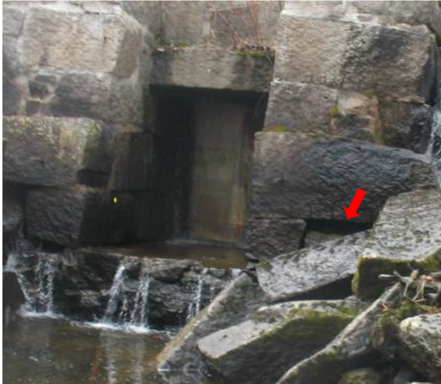
Photo 11. Downstream View of Closed Central Sluice Gate. Note Large Void in Masonry.
