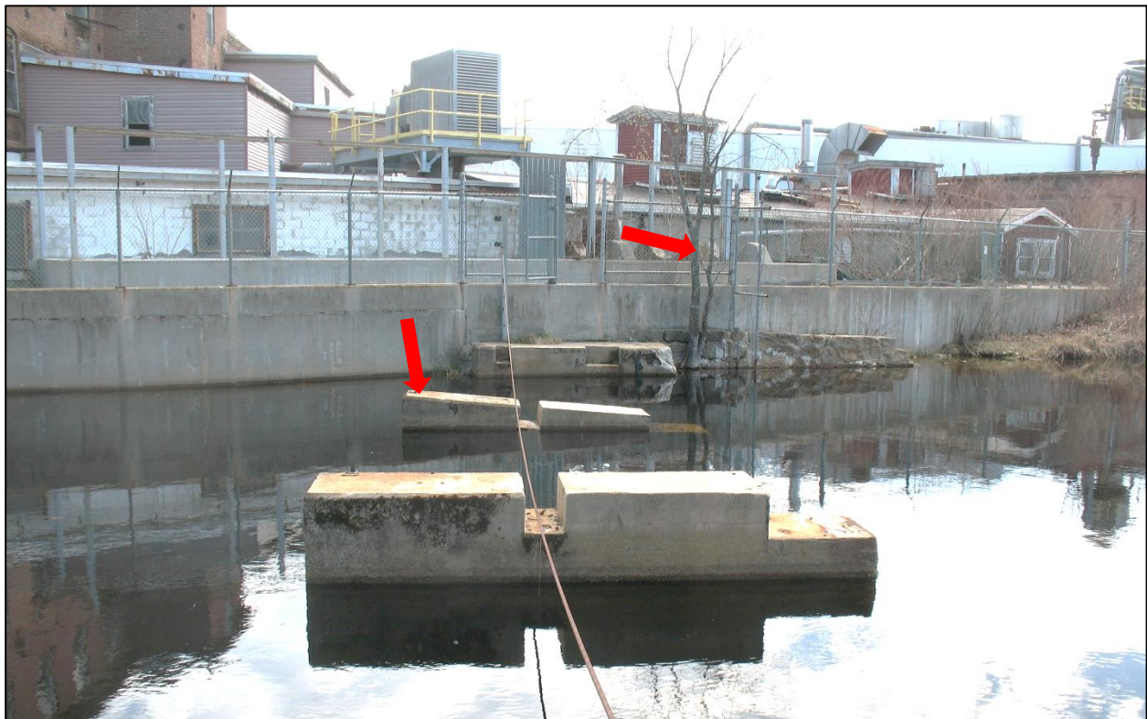
Photo 24. Right Approach Channel Retaining Wall and Old Piers Supporting Original Trashracks and Catwalk. Note Sagging Central Pier and Tree at Waterline.
