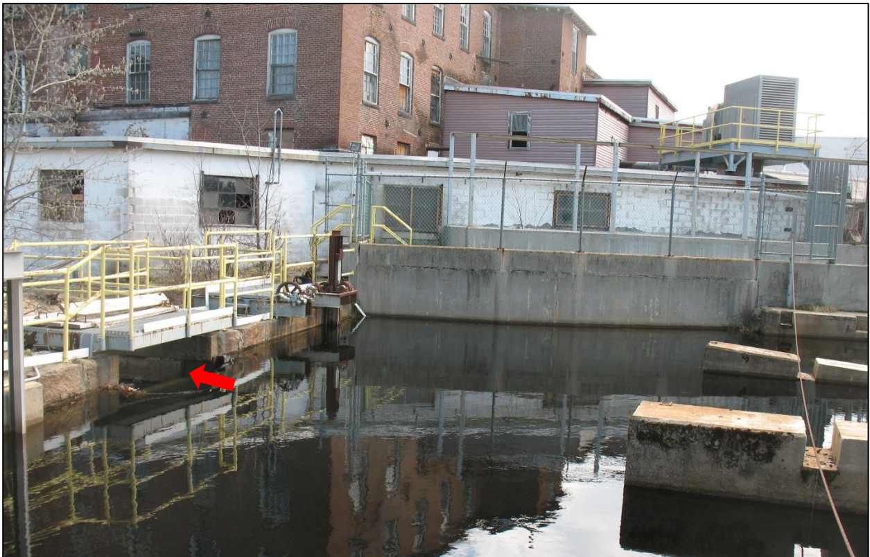
Photo 12. Upstream View of East Sluice.
