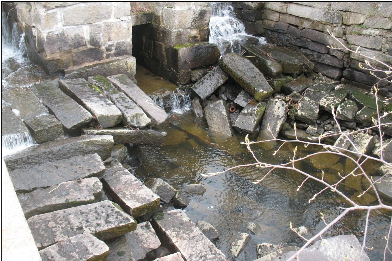
Photo 26. Disintegrated Stone Apron. Note Scour Hole at Dam Toe and in Channel Floor.
