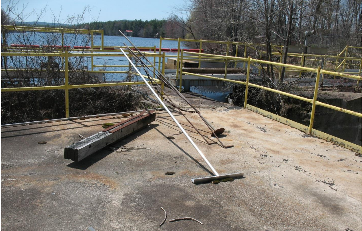
Photo 19. Concrete Dam Section Looking Upstream. Note Stored Lifting Rods Used for Stoplog Operation.
