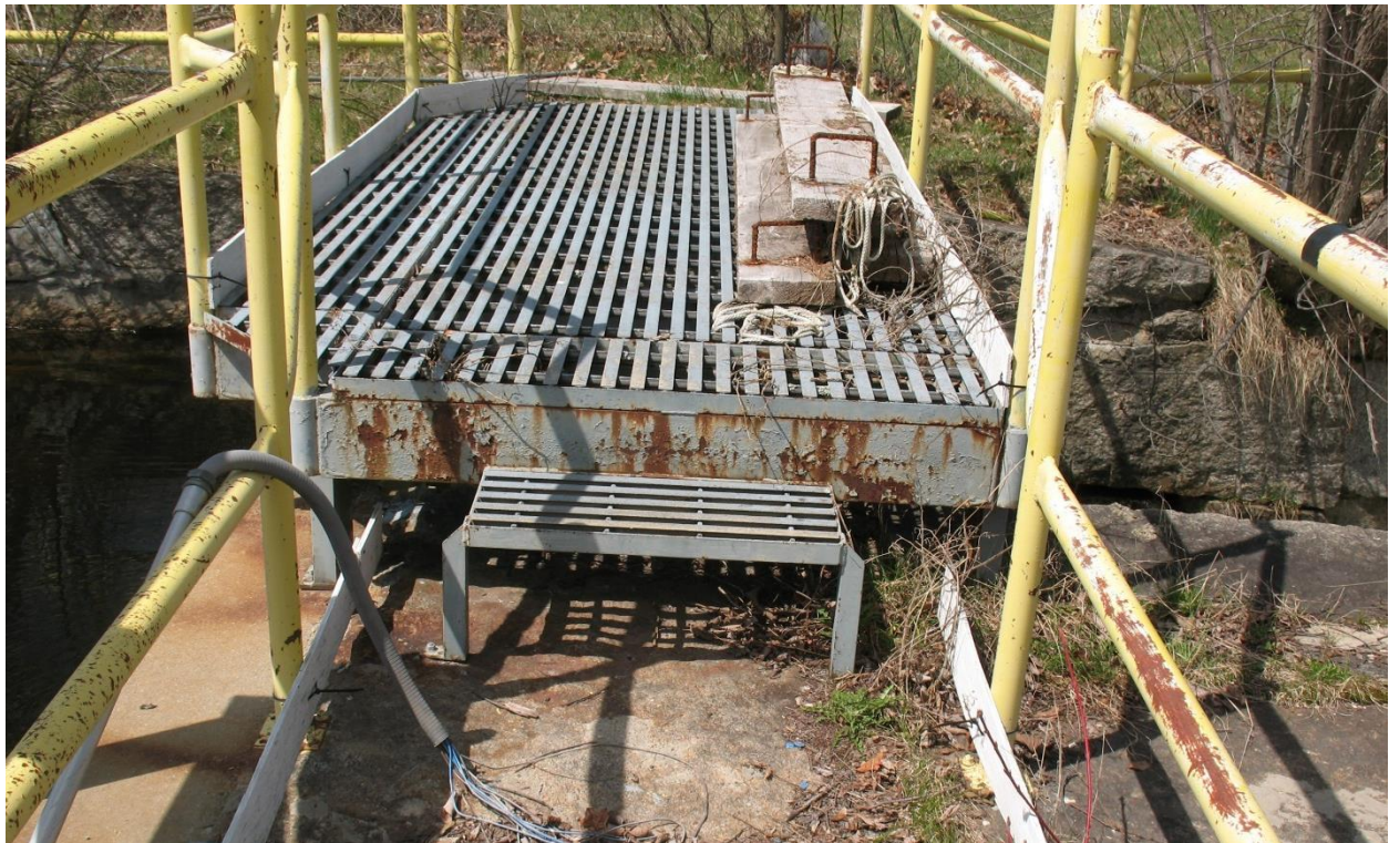
Photo 6. West Sluice Operating Platform.
