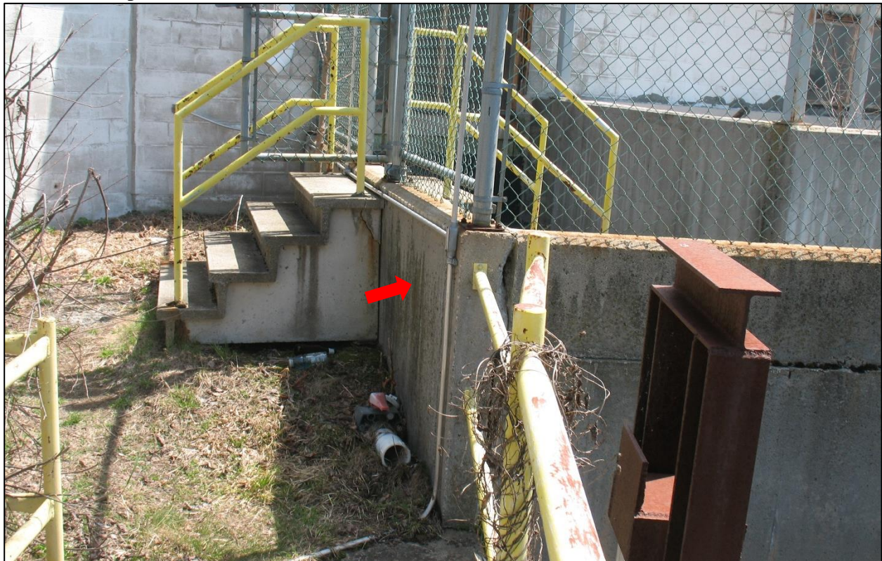
Photo 18. Concrete Dam Section at Mill Building and 3-foot High Concrete Parapet Wall (arrow) on Top of Dam.
