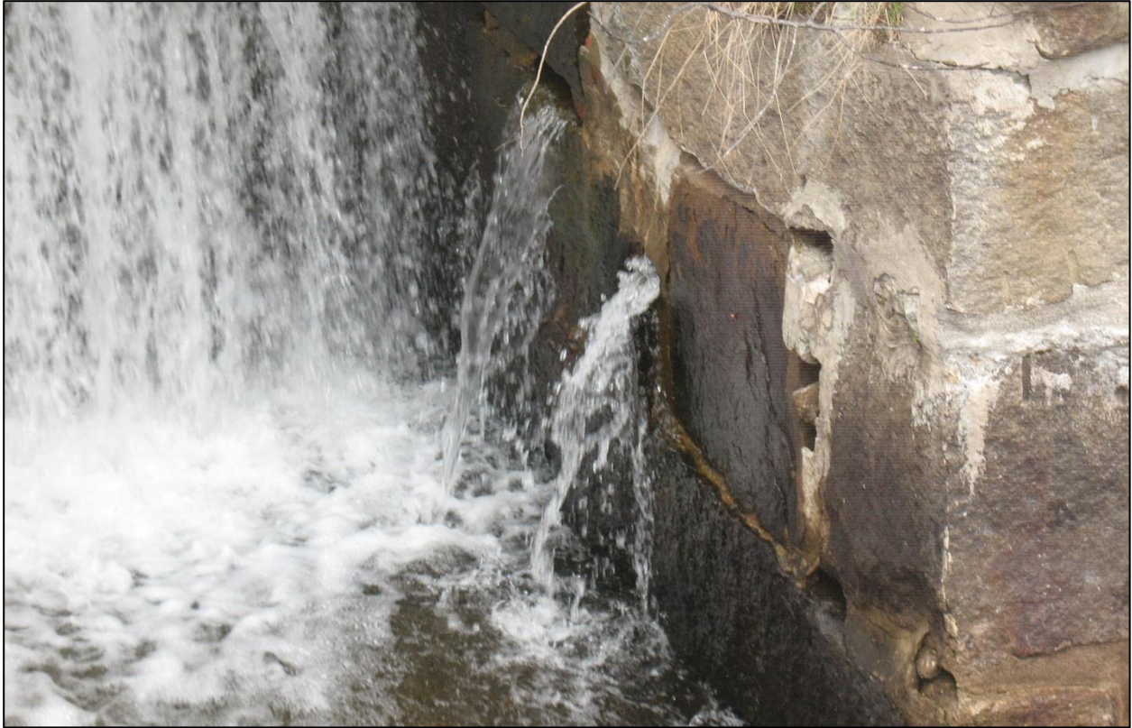
Photo 15. East Sluice Left Wall: Open Voids and Leakage in Masonry.
