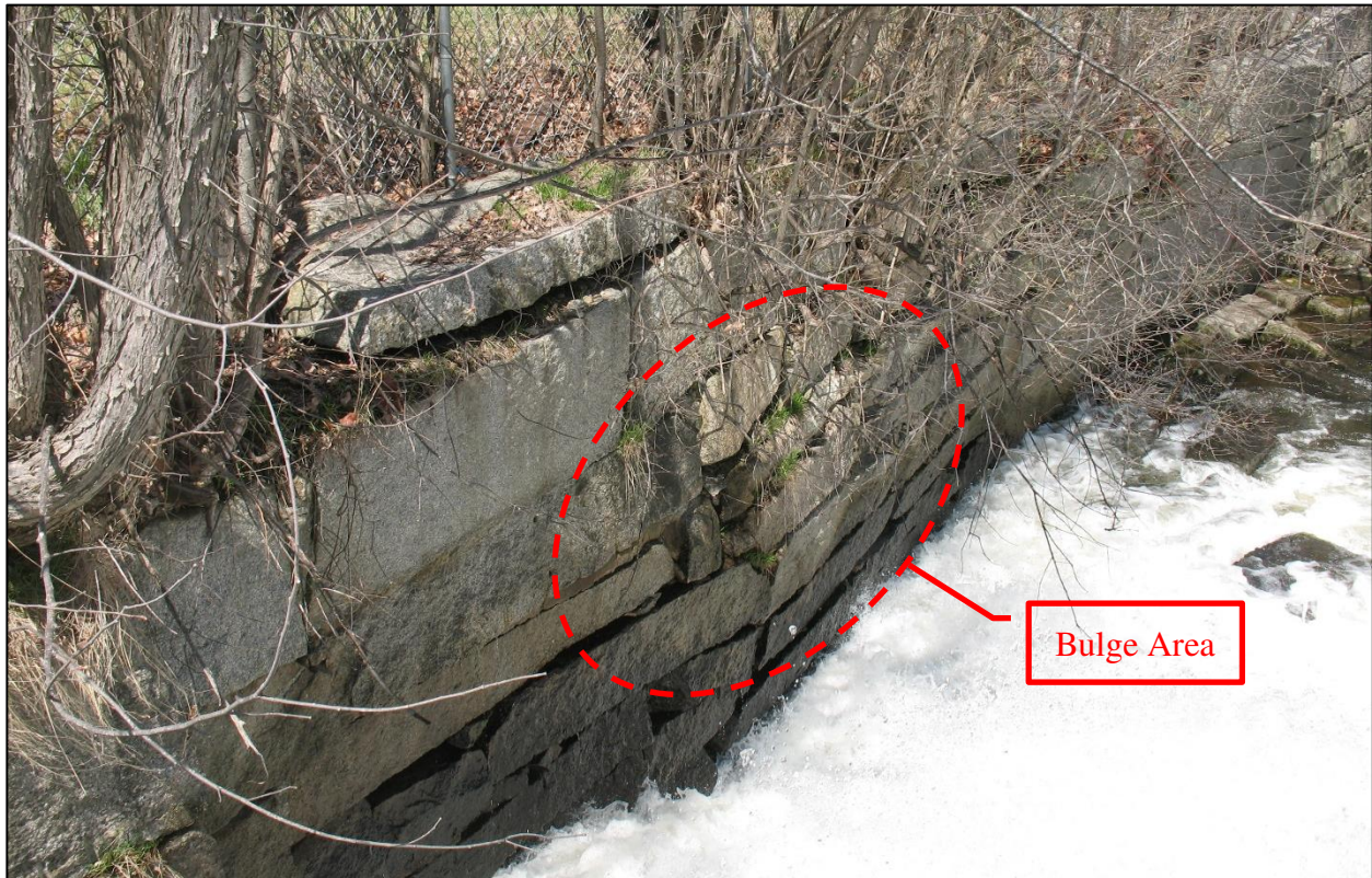
Photo 29. View of Left Discharge Channel Retaining Wall from Dam. Note Bulging, Displaced and Missing Stone, Voids, Large Trees and Brush.
