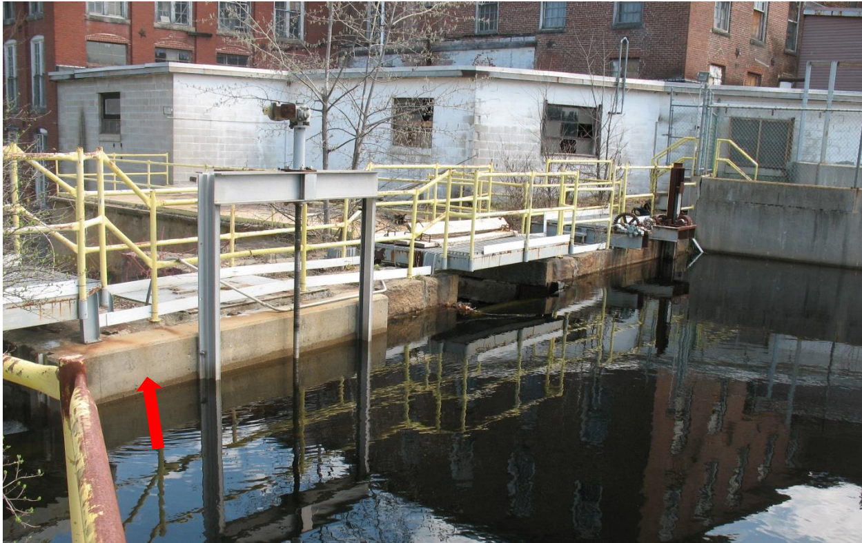
Photo 7. Upstream View of Central Sluice: Concrete Overlay (arrow), Gate Frame, Operator and Stem Installed in 1993.
