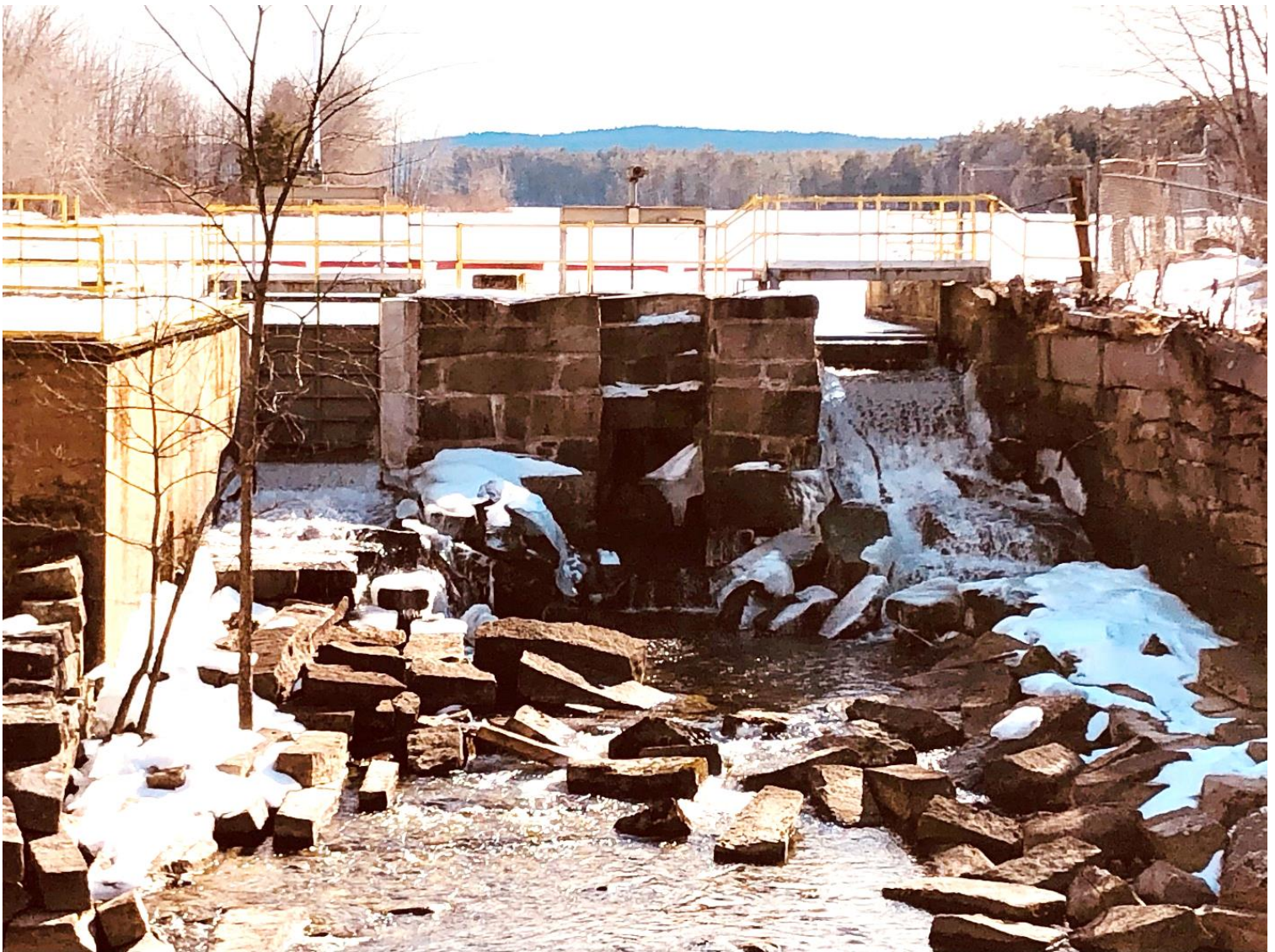
Oxford dam, March 2021. East gate is on the left.
