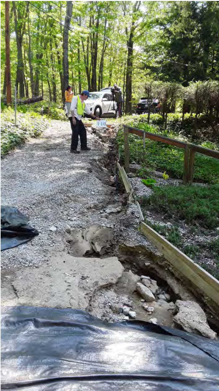
Site 1-10: High impact residential site. Large area experiencing gully erosion flowing directly into the lake without a buffer.
