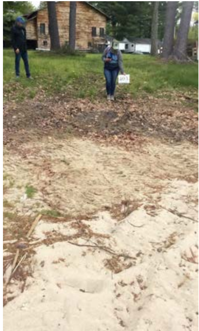
Site 4-03: A high impact commercial site. This site has identified gully surface erosion, shoreline erosion, and inadequate shoreline vegetation as primary problems.
