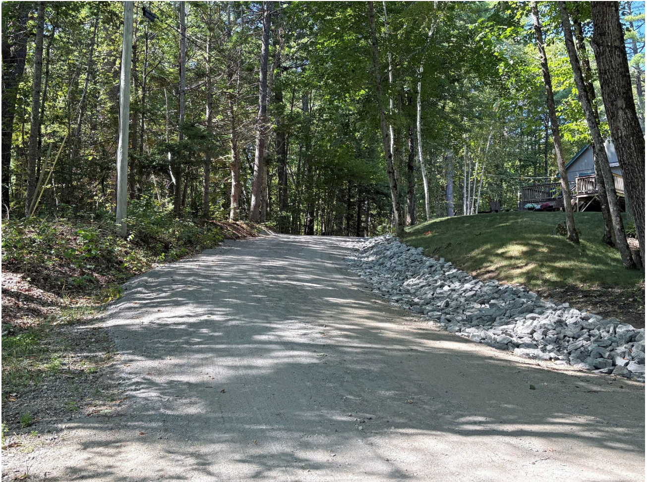
New road ditch and regrading at Wacipi Pines funded by 319 Grant Program
